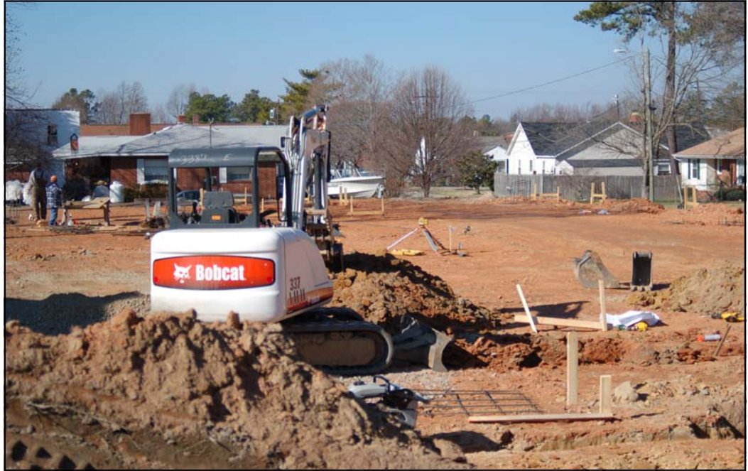
Construction has started on the 10 classroom building at Franklinton High School.
